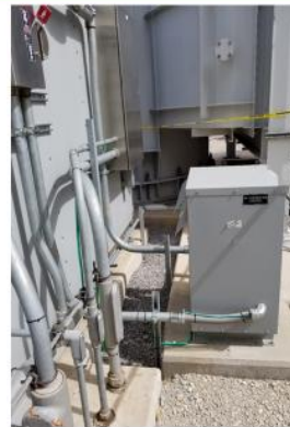
Outside a CEMS Shelter
